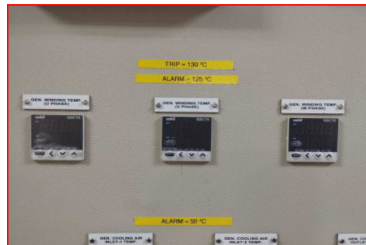
Temperature indicator for stator coils
