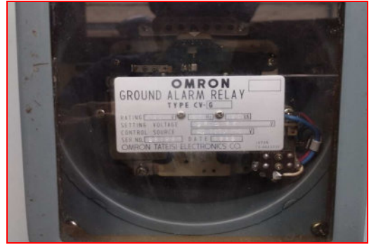
Ground over voltage relay
